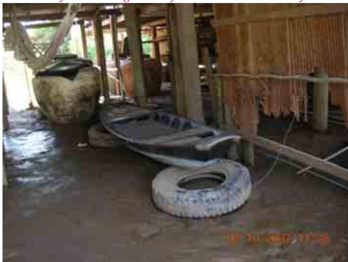
Large pots used for rain water harvesting. These houses can withstand floods as high as 11 feet. The boat is made of SS Steel.
